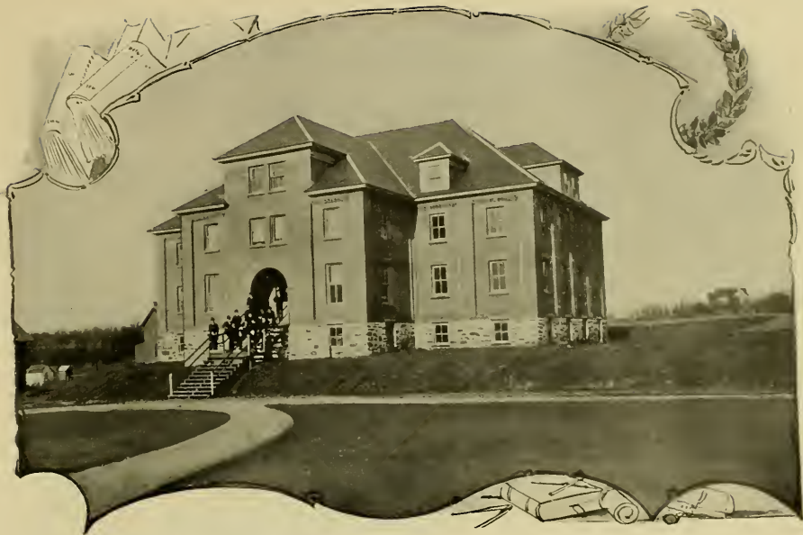
GYMNASIUM OF STATE NORMAL SCHOOL, EAST STROUDSBURG, PA., GEO. P. BIBLE, A. M., PRINCIPAL.
